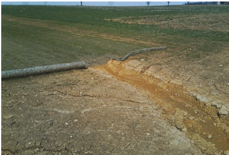
This farmer started using erosion control blanket on a newly constructed waterway, but didn't get it all secured before a heavy rain. You can see the amazing difference that the fabric makes.
