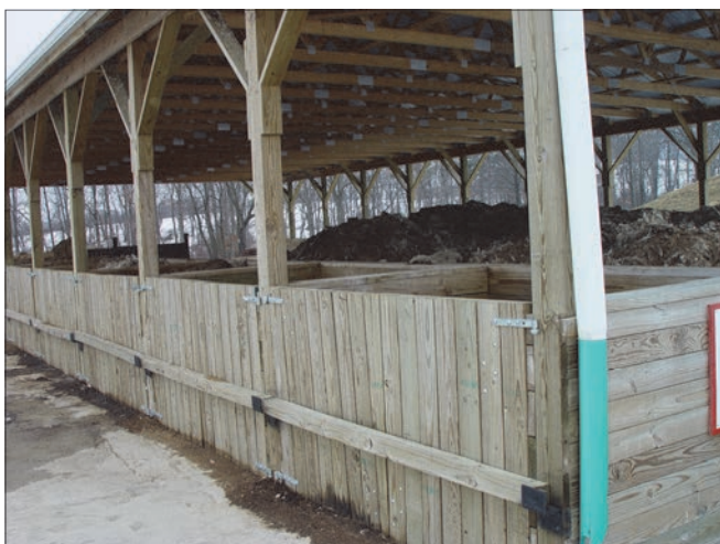
Mortality composting bins as part of roofed poultry manure stacking structures (above and right), using walls of treated lumber or concrete walls.
