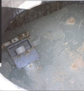
Milkhouse wastewater can be either pumped or siphoned from the concrete tank. Electric and pneumatic pumps are used to pump wastewater uphill or greater distances. Siphons can only be used when filter areas are located below the concrete tank.
