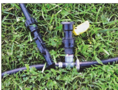
A frost free hydrant located in a pasture (right). At left, a quick disconnect for a water line where water trough portability is preferred.
