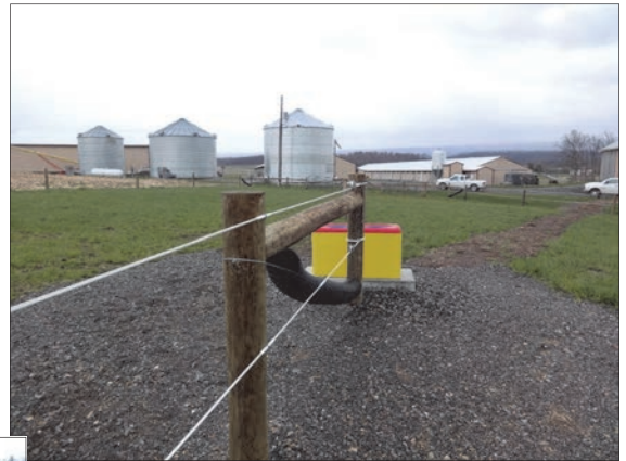
Reinforced gravel pads placed around newly installed water troughs and waterers at various beef and equine operations.
