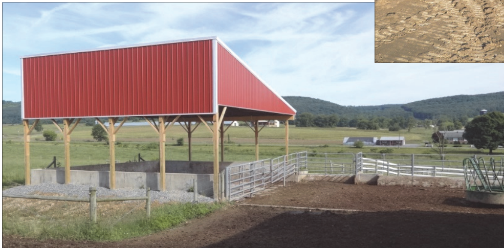
Roof installed over existing concrete manure stacking area for a beef barnyard.
