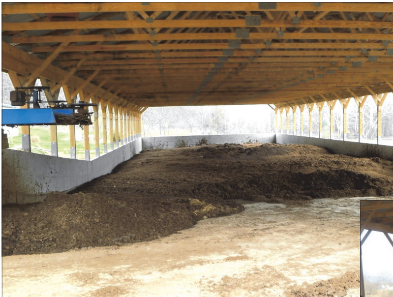
Roofed manure storages with concrete walls.
