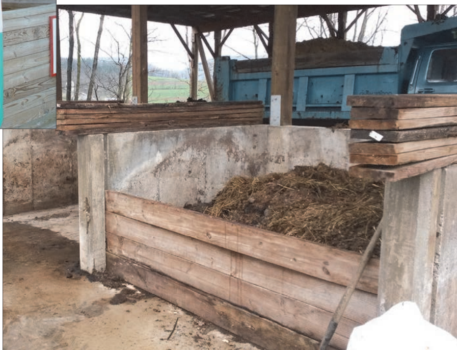
Mortality composting bins as part of roofed poultry manure stacking structures (above and right), using walls of treated lumber or concrete walls.
