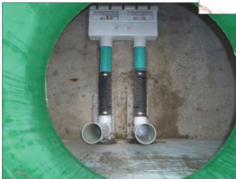
Milkhouse wastewater can be either pumped or siphoned from the concrete tank. Electric and pneumatic pumps are used to pump wastewater uphill or greater distances. Siphons can only be used when filter areas are located below the concrete tank.
