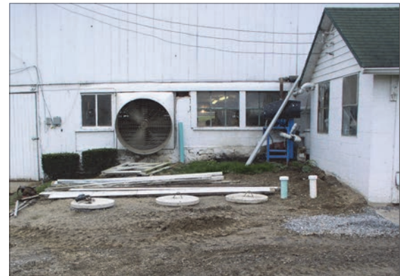
Concrete septic tanks being installed to intercept milkhouse wastewater at a dairy farm (right). The outlet goes to a vegetative filter area.
