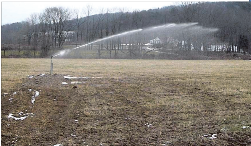
Irrigation provides another method of distributing wastewater in a vegetative area. The wastewater is pumped to the vegetative filter area where it irrigates the site through a spray nozzle. Wastewater can be sprayed on permanent pasture if it maintains lush vegetation.
